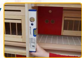
It must now be aligned using the spirit level and securely screwed to the back wall.
