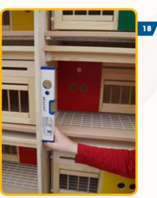
Then accurately align the box vertically and horizontally using a spirit level and securely screw it to the rear wall.
