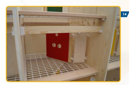
Fit the front bars into the plastic mounts on the side panels.
