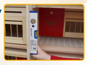
It must now be aligned using the spirit level and securely screwed to the back wall.
