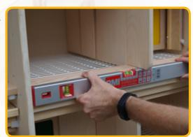
This must now be aligned using a spirit level and then be firmly screwed to the back wall.
