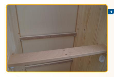
Press the beech wood perch bars onto the metal bolts on the upright side panels. 5 pieces per section. In doing so the notch on the bars must always point to the back.
