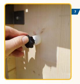
Screw on the mounting for the scraper blades (droppings blades). The white distance ring ensures that there is still clearance behind the droppings blade so that the dust and dirt cannot collect behind the scraper blade.
