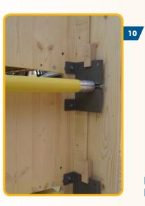
Fit the panel for the return side to the bearing plates.
